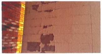
Spalling was noted on the exterior concrete block texture.
