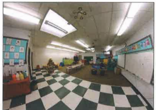
The school has a large central core of instructional spaces with no natural lighting or ventilation.
