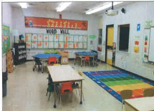
There is a lack of break out spaces and small group work areas. An existing classroom is used to provide areas.
